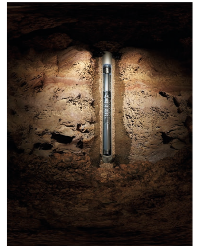
Pumping the water up requires sturdy systems
