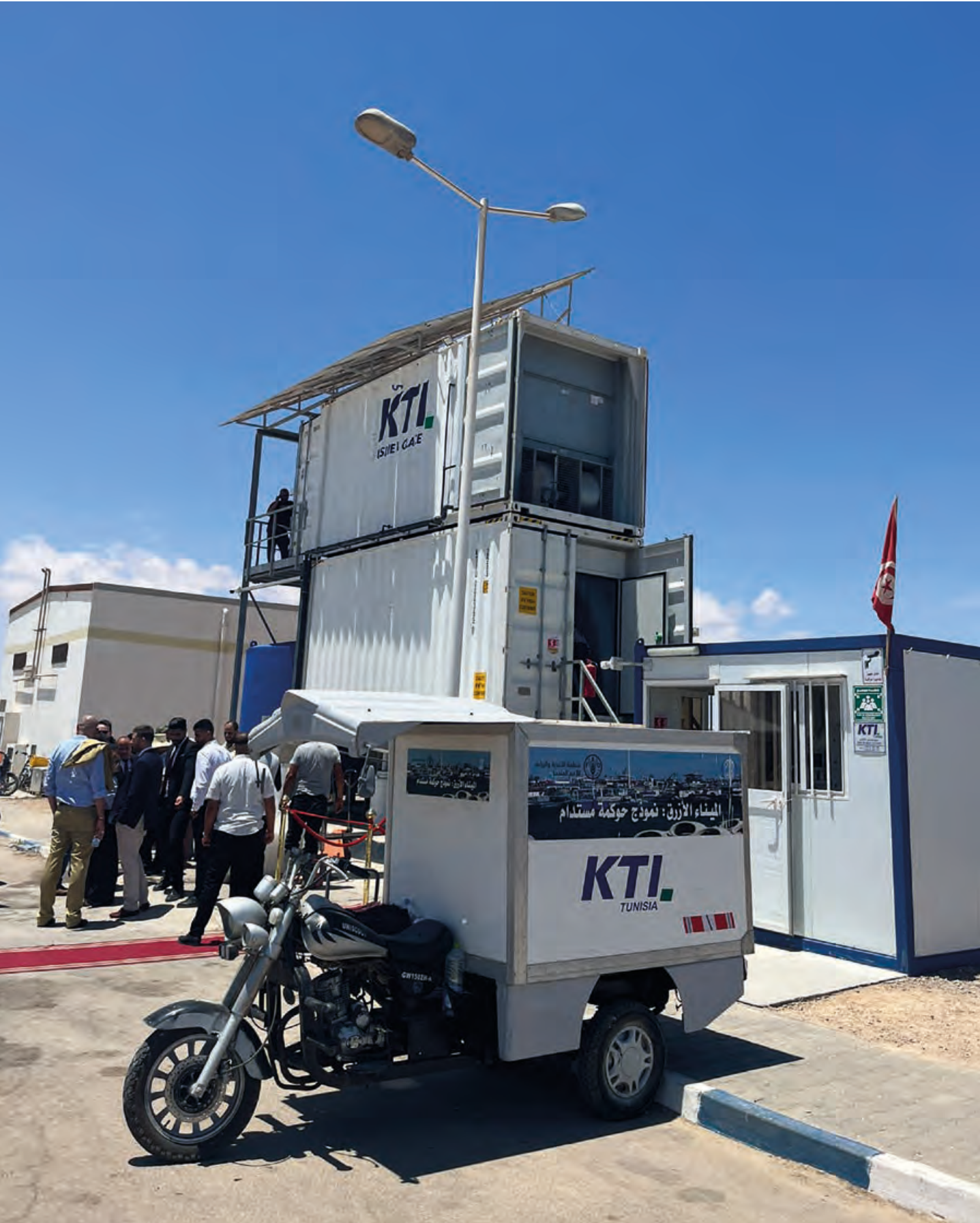
KTI ice plant at Zarzis harbour, Tunisia
