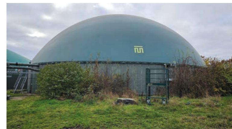
Biogas production in a real-world setting
